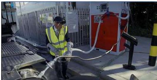
Place the filling hose back in its holder by the main control panel.
